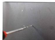
4 Drill holes into the drywall and insert the drywall mounts.
