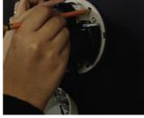
3 Use camera mounting template or your camera to mark the holes as required.
